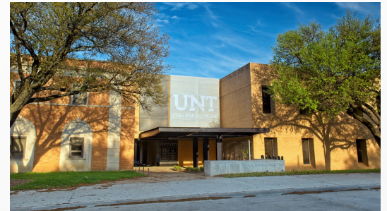
Paul Voertman Concert Hall UNT Music Bldg 415 Avenue C, Denton, TX 76201
