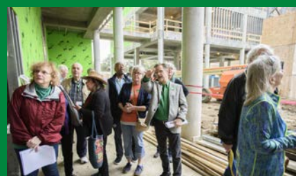
Tour of UNT CVAD renovations
