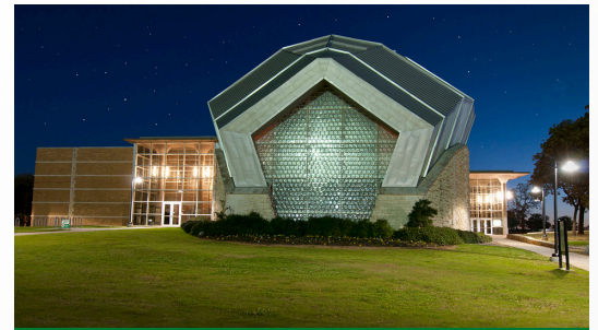
Murchison Performing Arts Center 2100 North I-35, Denton, TX 76201
